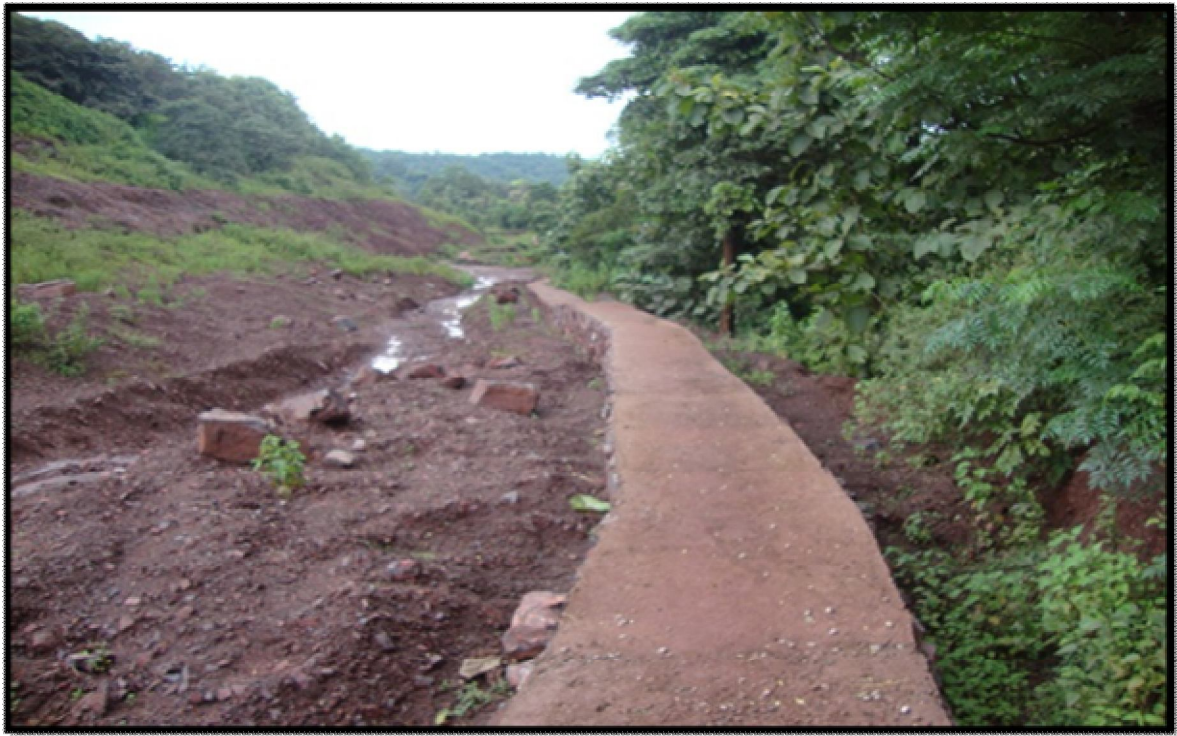
Photo 1 – Retaining Wall constructed at the base of sub-grade dump
