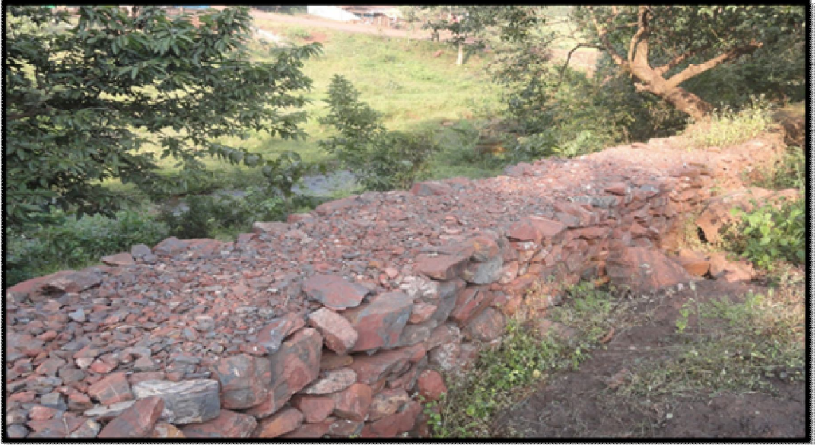
Photo – 3 – Photo showing the provision of guard wall all along the Nallahs
